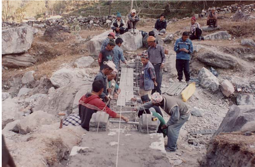
15. Walkway erection
