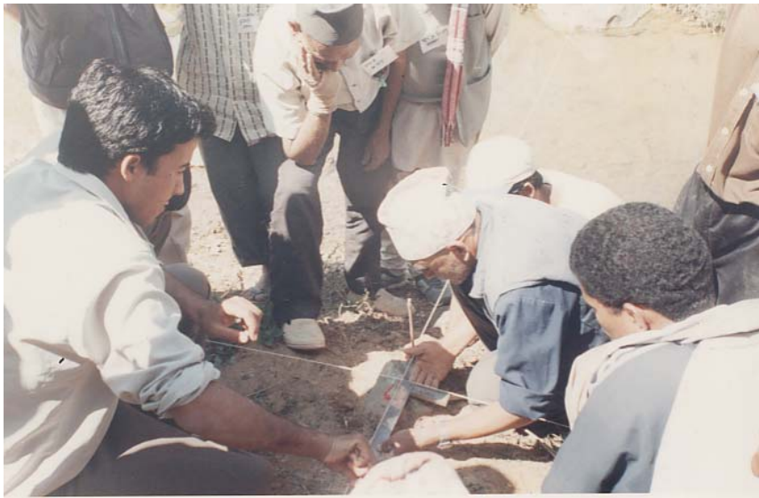
5. Centre Line Fixing
