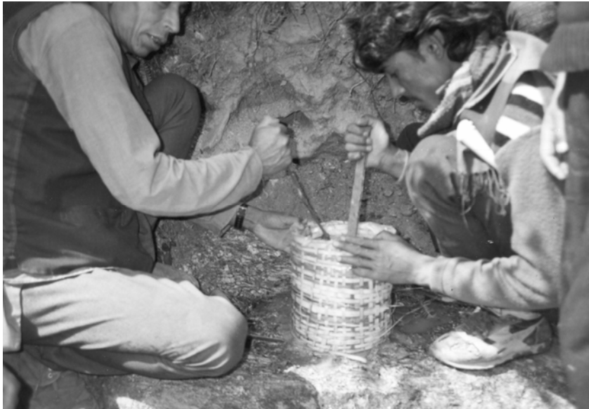
10. Cement for drum anchor
