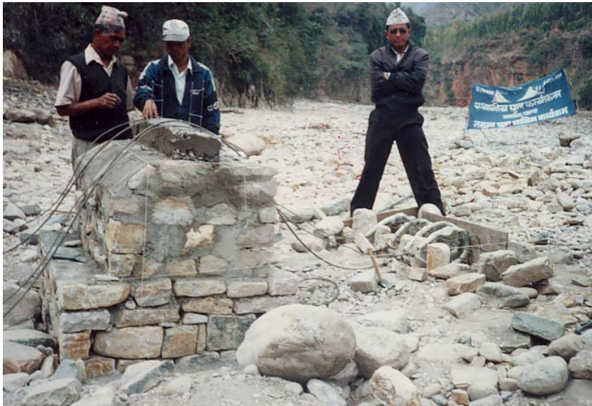
11. Tower with WWC saddle concreting
