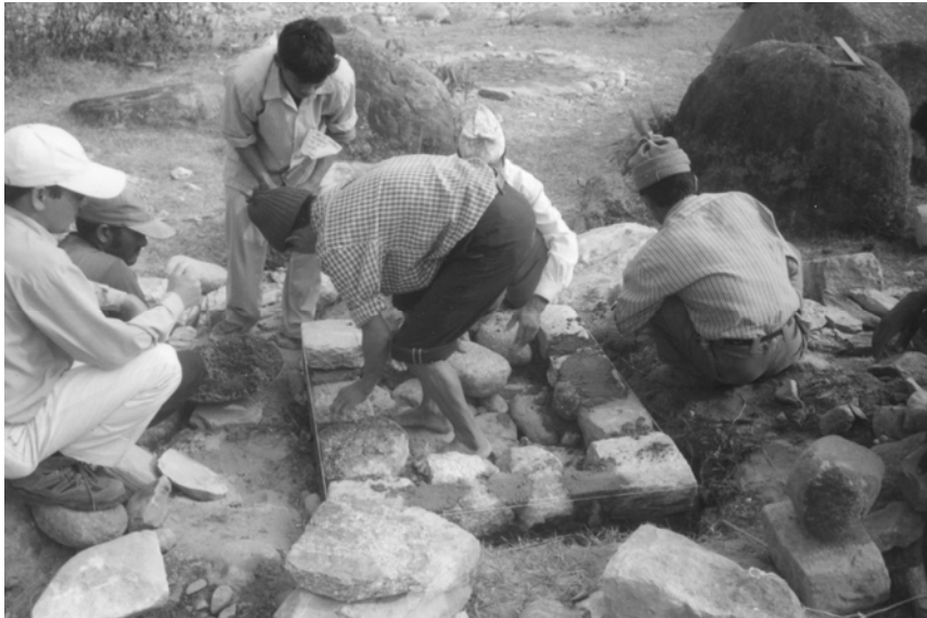
7. Cement stone masonry on 1:1 stone block's tower base
