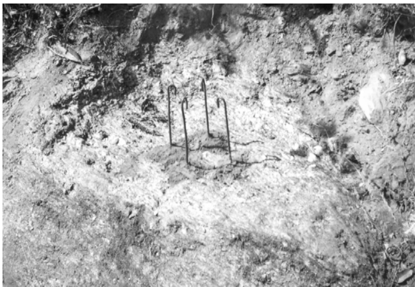
9. Grouting vertical rods in rock holes for drum anchor
