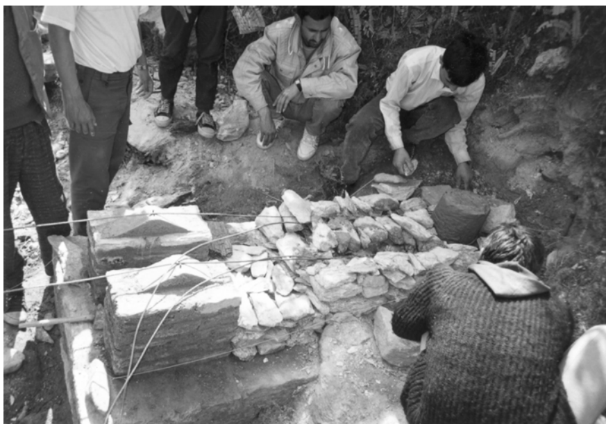
14. Concrete for cable covering
