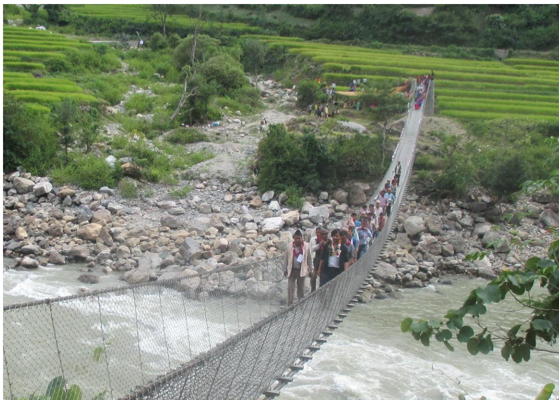
Raikar trail bridge has replaced the previous tuin that existed across Photo: Indra DC (RTAP-SEBAC/Nepal)
