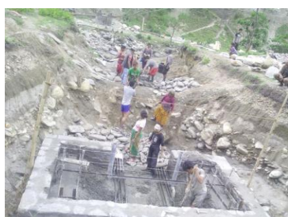
Jhangrali Trail Bridge (Dolakha) damaged by the earthquake under reconstruction
