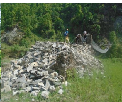
Maminlung Trail bridge damaged by earthquake (Rasuwa)
