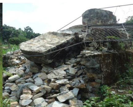
Katahare Trail Bridge damaged by earthquake (Dhading)
