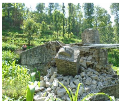
Katunje besi Ranitar trail bridge damaged by earthquake (Sindhupalchok)
