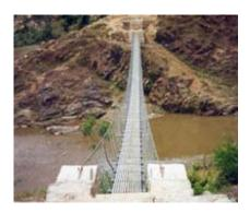
Since 2002, after the proven observations, Manuals on Suspended and Suspension types of SSTB Bridge are developed and published. SSTB type of bridge is to be designed for spans of up to 120 meters. The walkway width is 70 cm or 106 cm for suspended and 106 cm for suspension type bridge.
